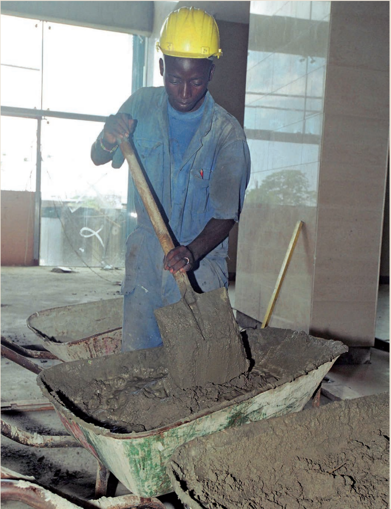
A bricklayer on a construction site in Dar es Salaam, United Republic of Tanzania. The construction industry is another sector in which self-employment and free-lance work has become more common.
